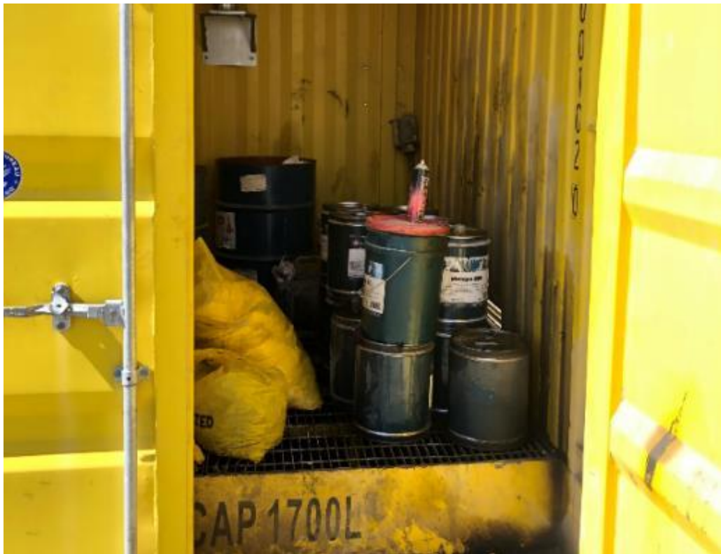
Figure 14: Storage of oils within bunded containers
